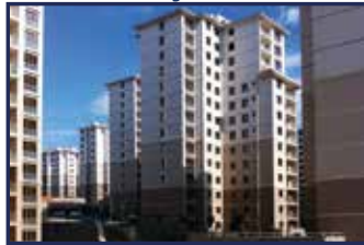
Tuzla Estate Housing
